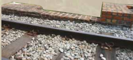
Railway tracks dividing Mukim 5 & 6
